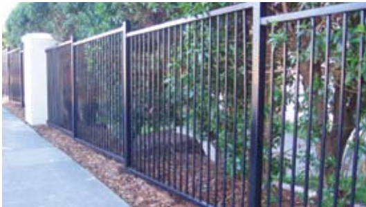
New fencing complete along portions of 19th Avenue
